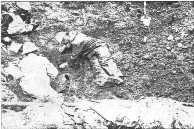
Figure 2. Crews work to forensically uncover ruptured pipeline.
