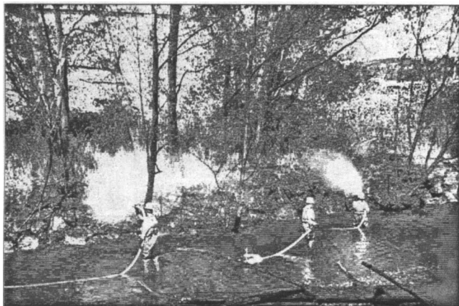
Figure 3. Float-a-pumps used low pressure to wash the banks and high pressure to spray streambeds.
